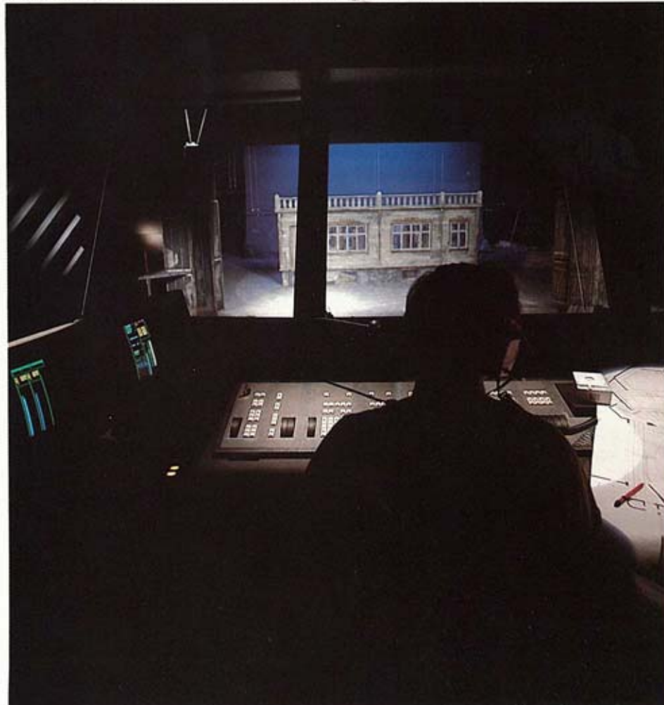
ADB equipment is installed in the lighting control rooms situated at the rear of the main theatre.
